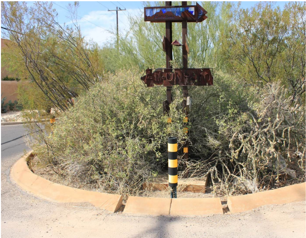
A curb cut in Dunbar-Spring that, come rain, directs stormwater to a planting. Photographer: Chris Malloy/Bloomberg
