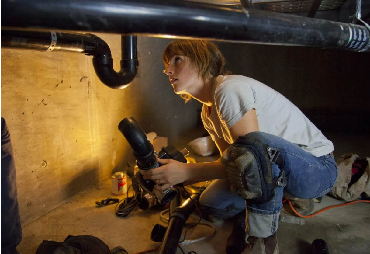
A diverter valve for a greywater system is installed at a new home construction site in Los Angeles. A branched greywater system diverts discarded water from sinks and washing machines away from sewage lines, and recycles it back via a gravity-fed drain system for irrigation and back into the aquifer. Photographer: Citizen of the Planet/Education Images/Universal Images Group via Getty Images
